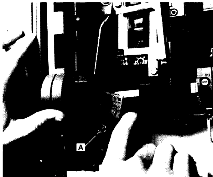
Figure 39. Operating handle and door interlocks.
