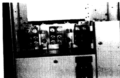
Figure 2. Isolating panel allows access to main and vertical bus joints.
